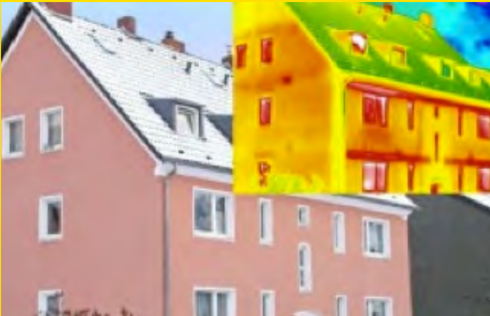
Thermal bridging leading to heat loss (the red parts of the image) can be seen in an infrared photo
