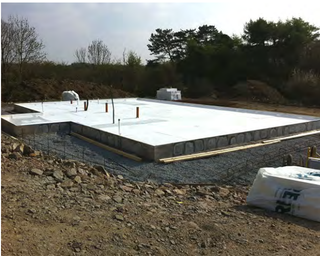
This load bearing insulated foundation system helps eliminate thermal bridging from foundations. Image courtesy Kore Systems
