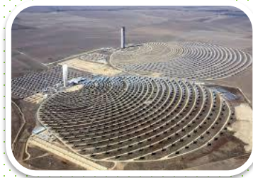
Solar thermal Power plants
