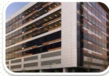
Aluminium glass facades
