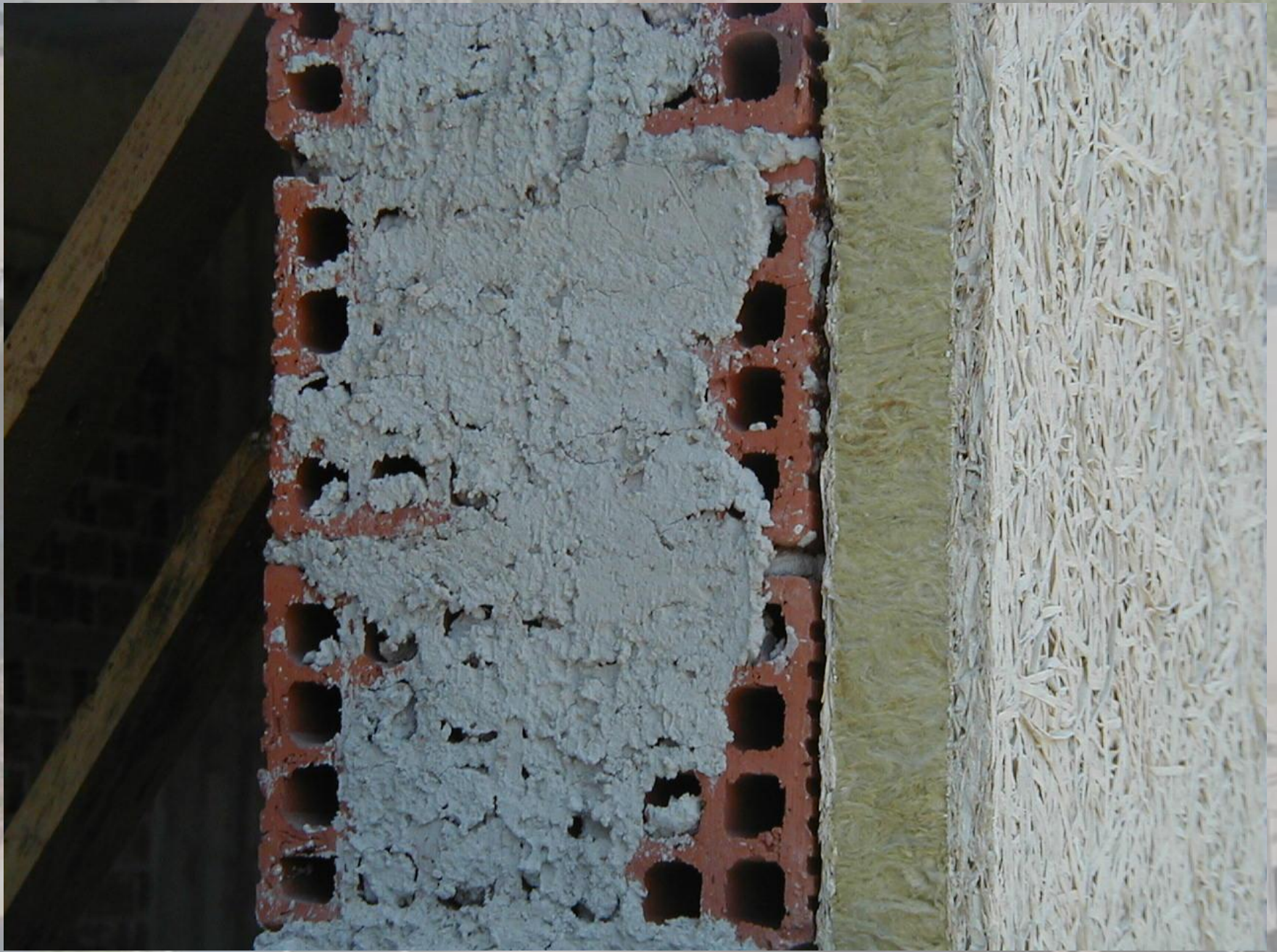
Detail of external brickwork with external insulation
