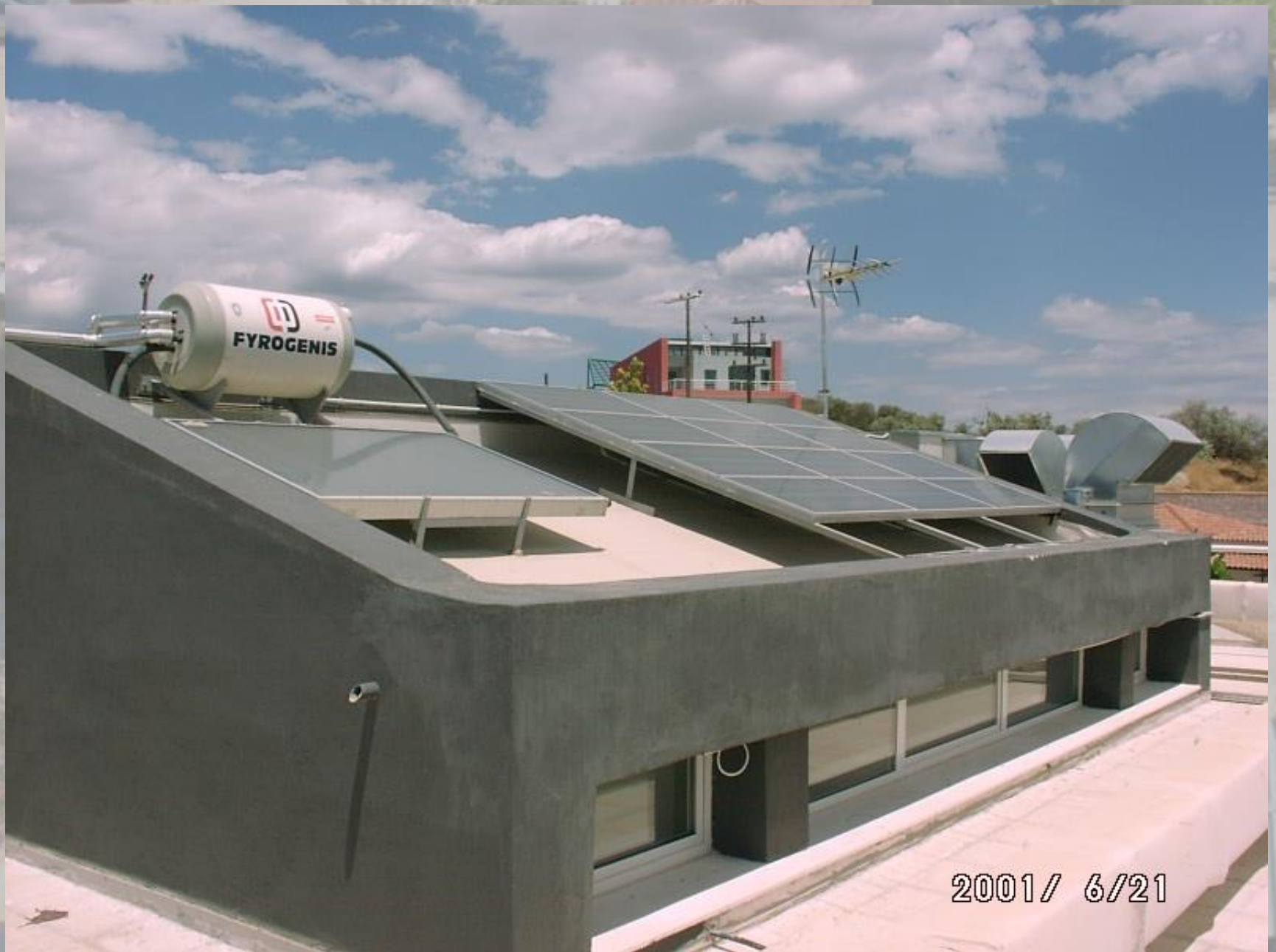
P/V 600W on the sloping part of the roof.
