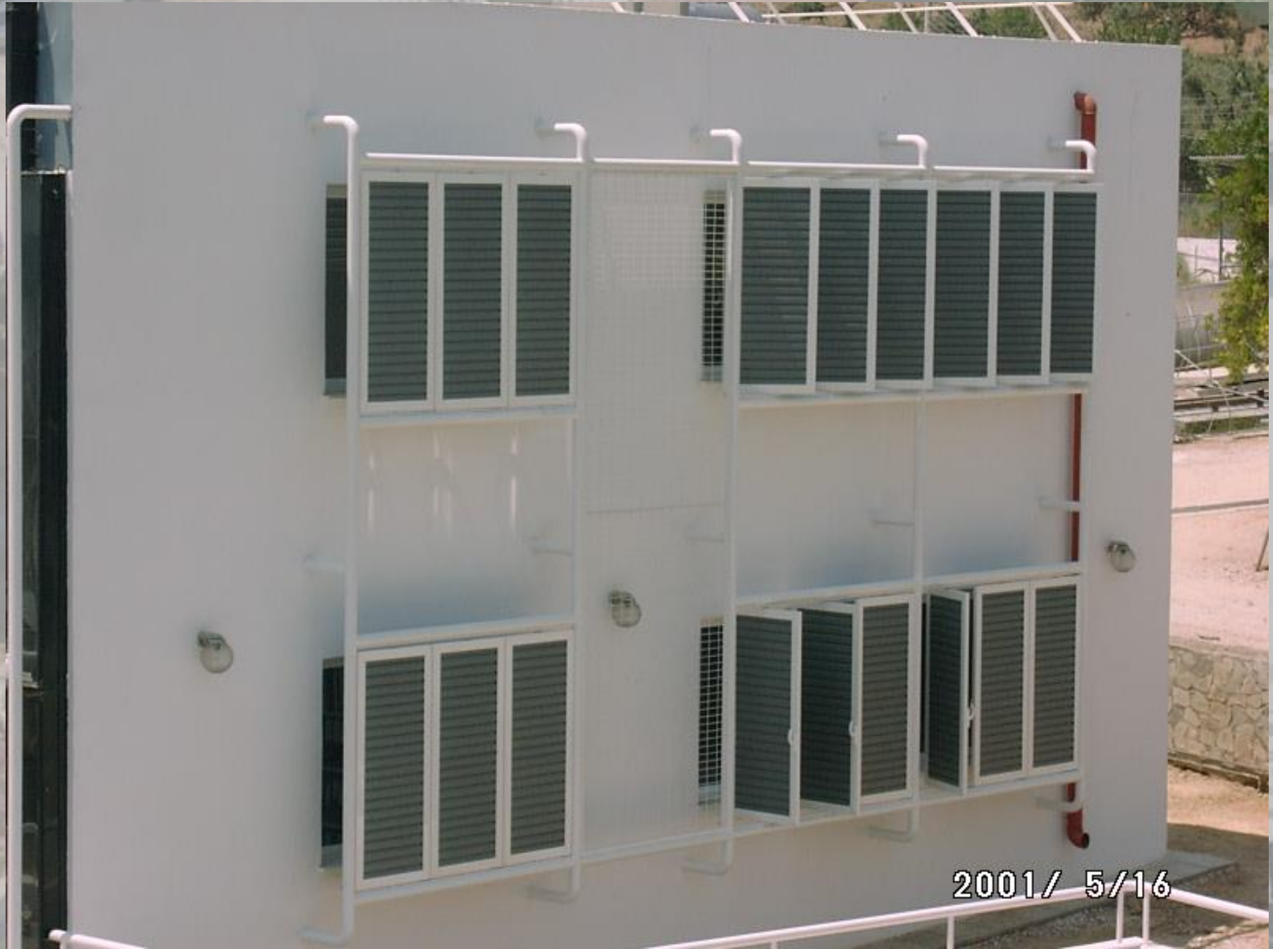
Sun protection system on the east & west facades
