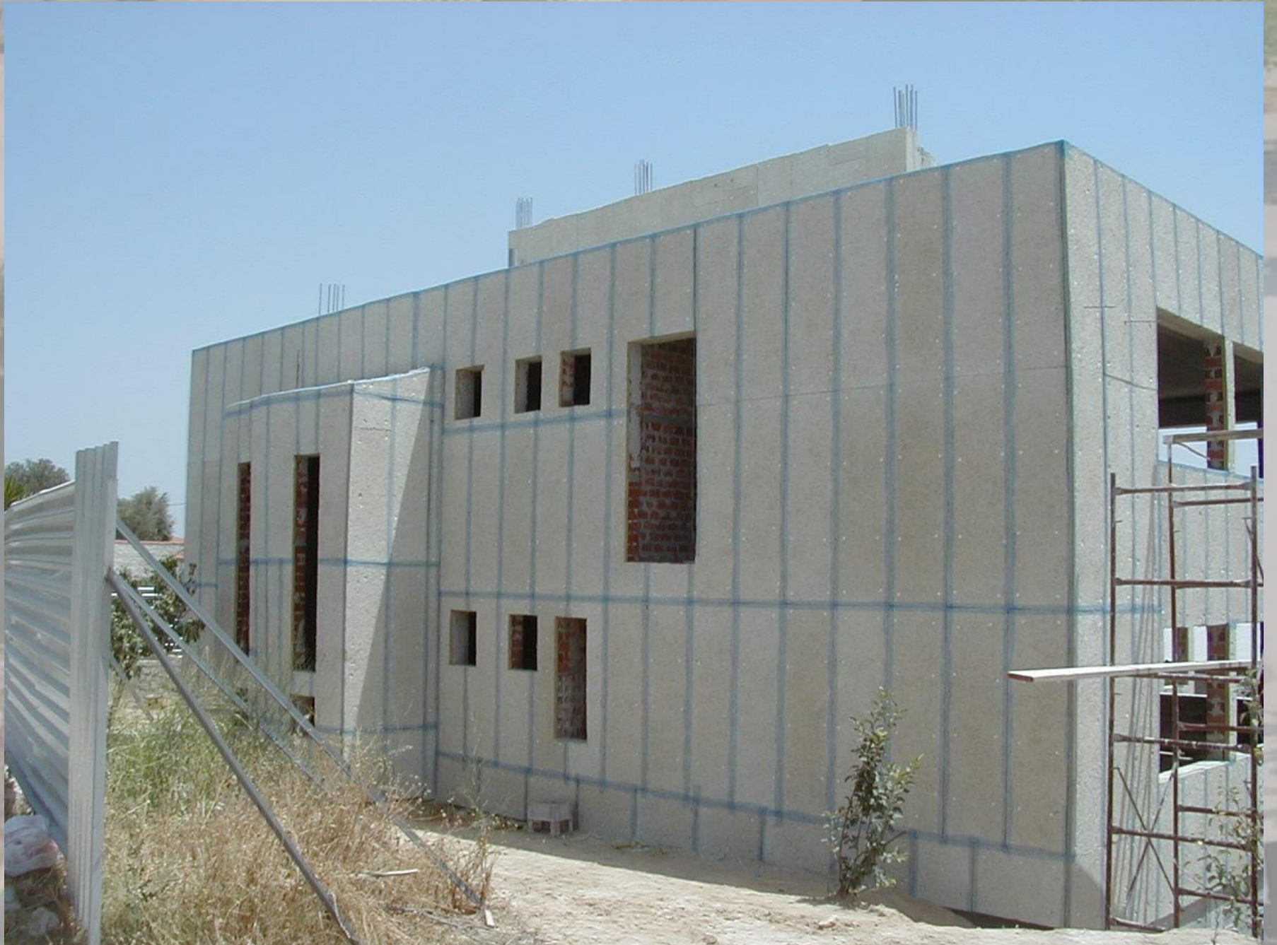
External insulation on the north face of the building
