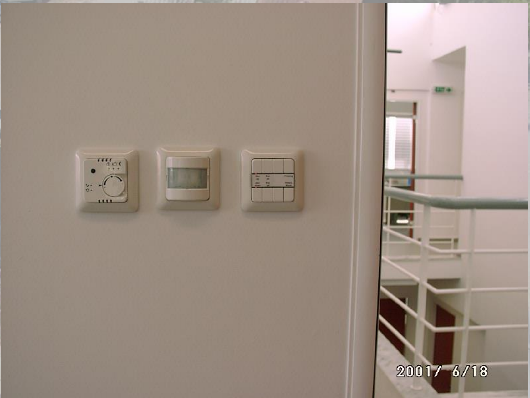
Room thermostat, occupancy sensor and eight function switch installed throughout the building's rooms.
