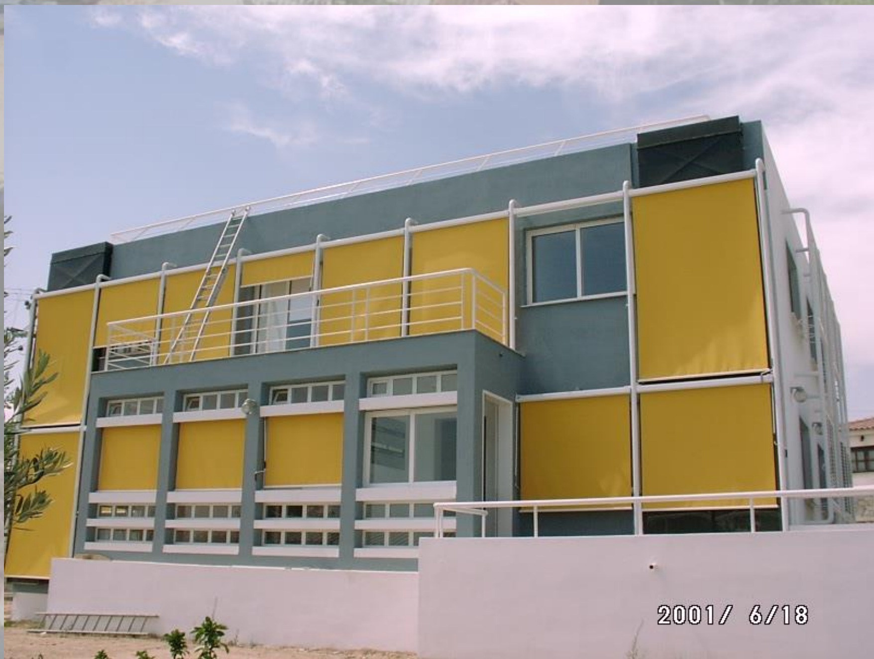
Sun protection system on the south facade
