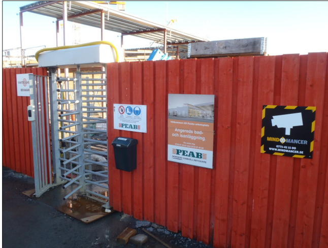
Figure 3.9. The use of access passes is expected to be adopted in Finland. This picture shows a staff entrance in Sweden where entrance gate posts are already used to monitor who is entering a worksite. Access control may also be used to prevent the use of clandestine workers.
