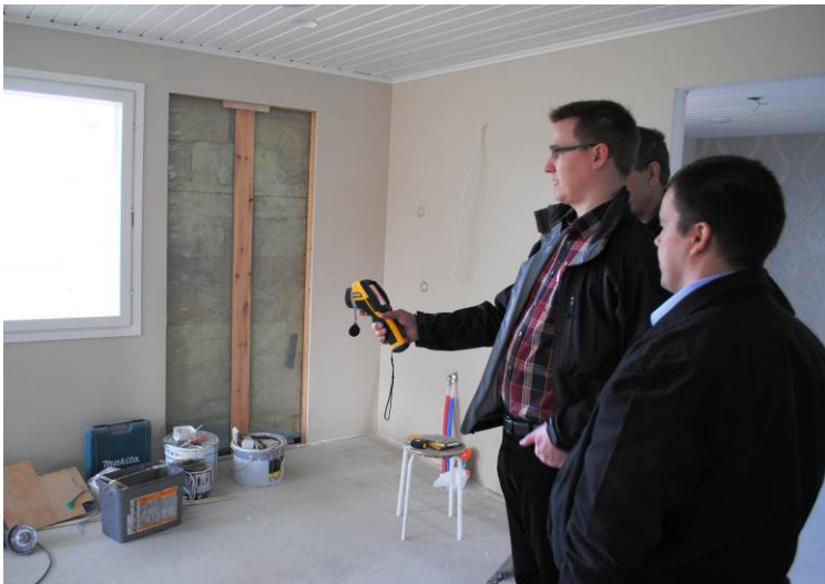
Picture 9: A building's airtightness is essential from the standpoint of energy efficiency. Air leak locations are observed with a thermographic camera at a Build Up Skills workshop in May 2012.
