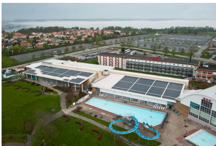
Figure 5.21 Rosenlundsbadet solar cells on roofs in Jönköping.
