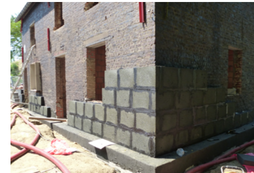
Insulation works. © ThInk E
