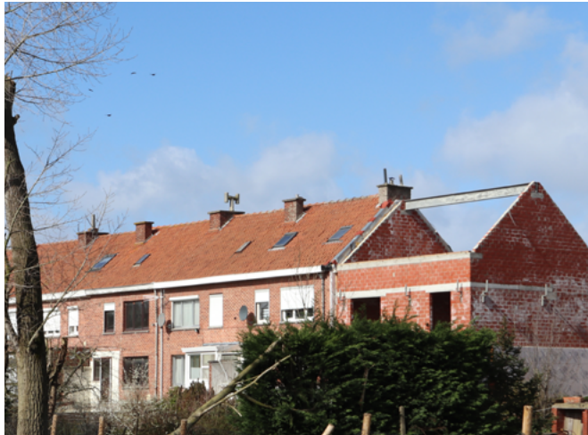
Retrofitting project in Kortrijk, Belgium © Agata Smok
