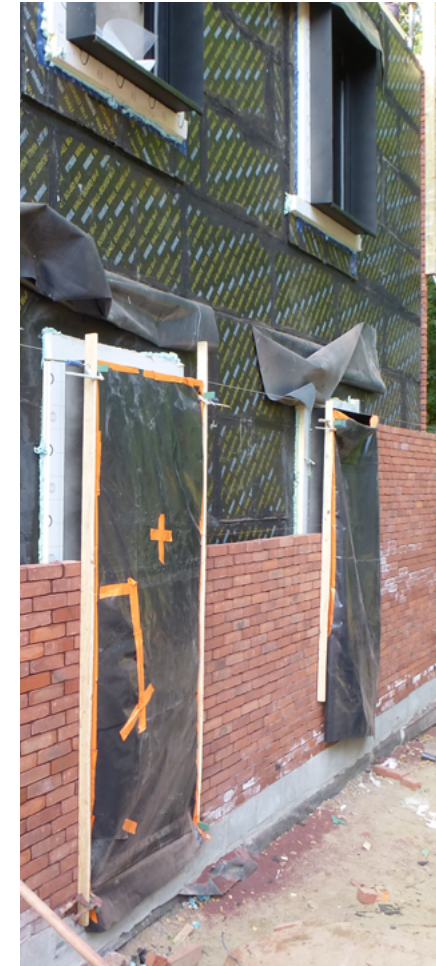
Retrofitting works . © Smart Cities Marketplace
