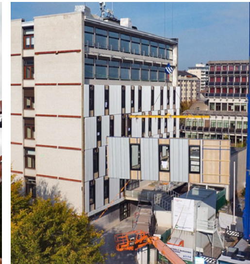
Energy-efficient façade renovation works for CRAC office building in Namur, Belgium © Machiels Building Solutions 2019
