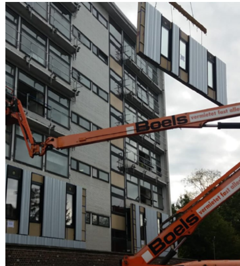
Energy-efficient façade renovation works for CRAC office building in Namur, Belgium © Machiels Building Solutions 2019
