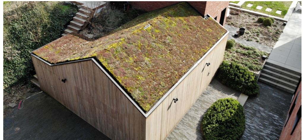
Green roof in Oud-Heverlee, Belgium STORY Horizon 2020 Demo Site. © ThInk E
