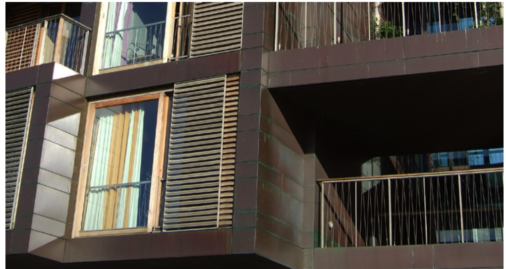
External shading integrated into the architecture of the building: overhangs, mobile louvres (Tietgencollegiet, Copenhagen). © Smart Cities Marketplace
