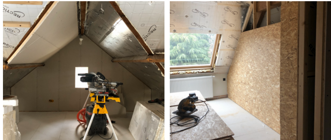
Attic insulation works in a single-family house in Belgium © Agata Smok
