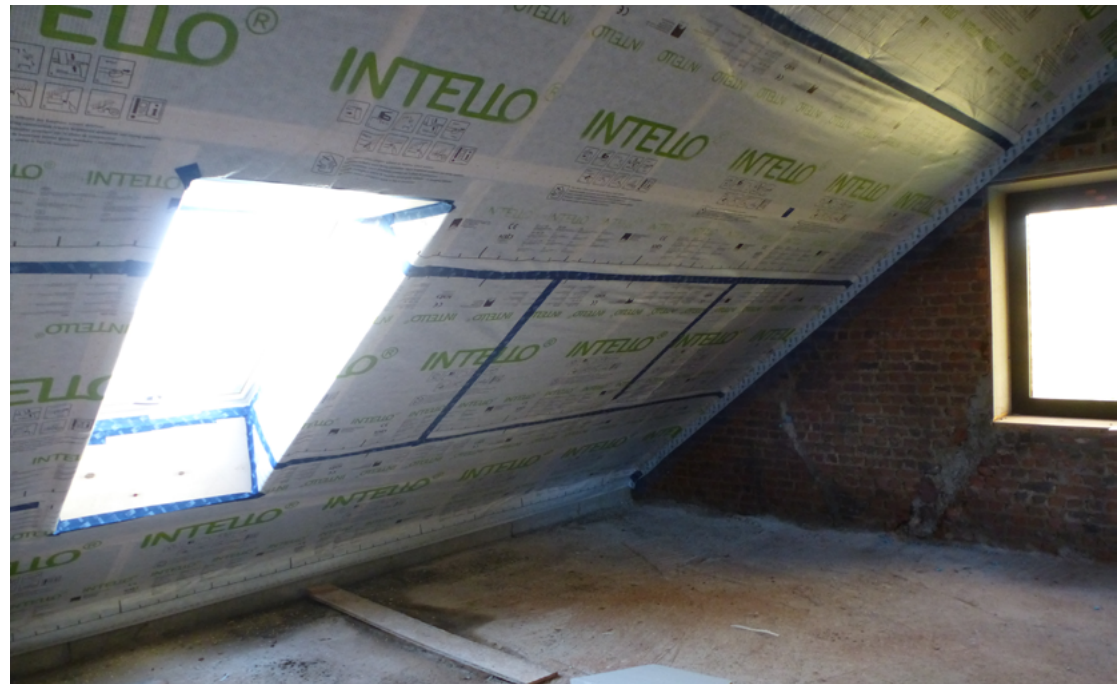
Retrofitting works . © Smart Cities Marketplace
