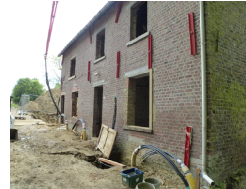
Situation before insulation. © ThInk E
