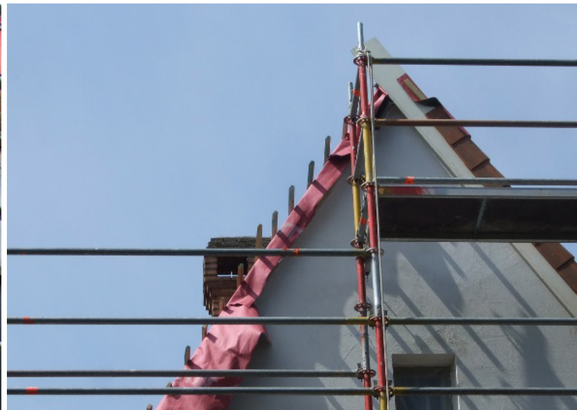
Illustration of the need to redesign building nodes, e.g., where retrofitted roof and façade meet. © Smart Cities Marketplace
