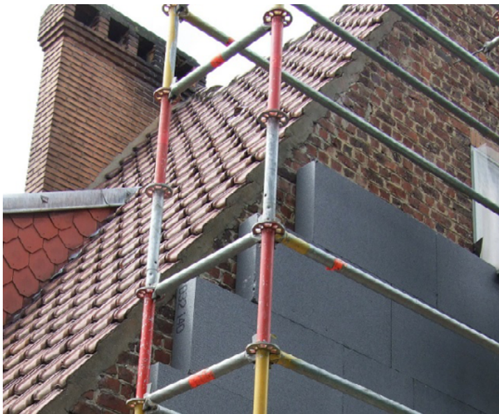
Illustration of the need to redesign building nodes, e.g., where retrofitted roof and façade meet. © Smart Cities Marketplace
