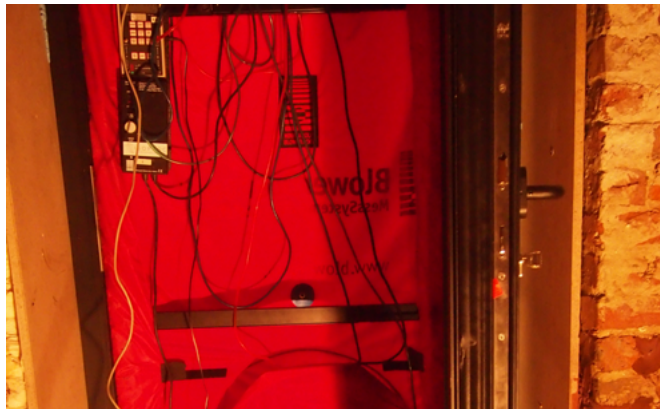
Blowerdoor test. © Th!nk E
