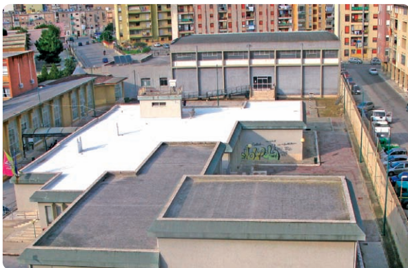
Figure 13. The building in Trapani application of the cool paint
