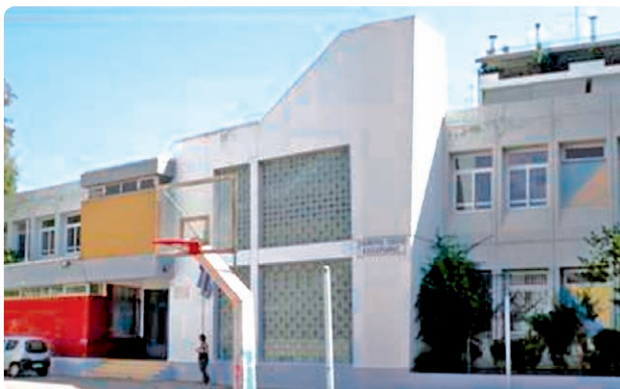
Figure 5. School building in Kaisariani, Athens, Greece
