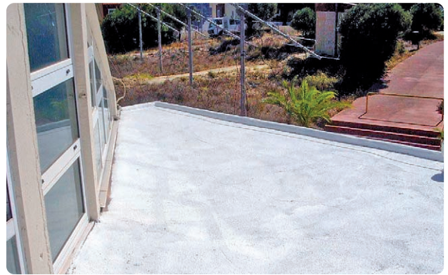
Figure 10. The roof after the cool coating was applied
