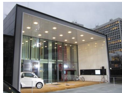
EFFICIENCY HOUSE PLUS (BERLIN): A PILOT PROJECT OF THE GERMAN BUILDING MINISTRY © FRAUNHOFER
