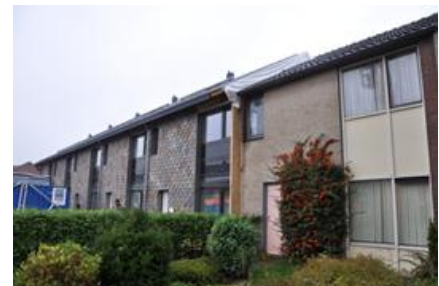
PASSIVE HOUSE RENOVATION AT THE KROEVEN (ROOSENDAAL, NETHERLANDS) © FRANK HANSWIJK
