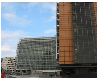
Photo of the Berlaymont building; headquarter of the EU Commission in Brussels. The façade of the building features glass slats that can be arranged similar to a double glazed façade.
