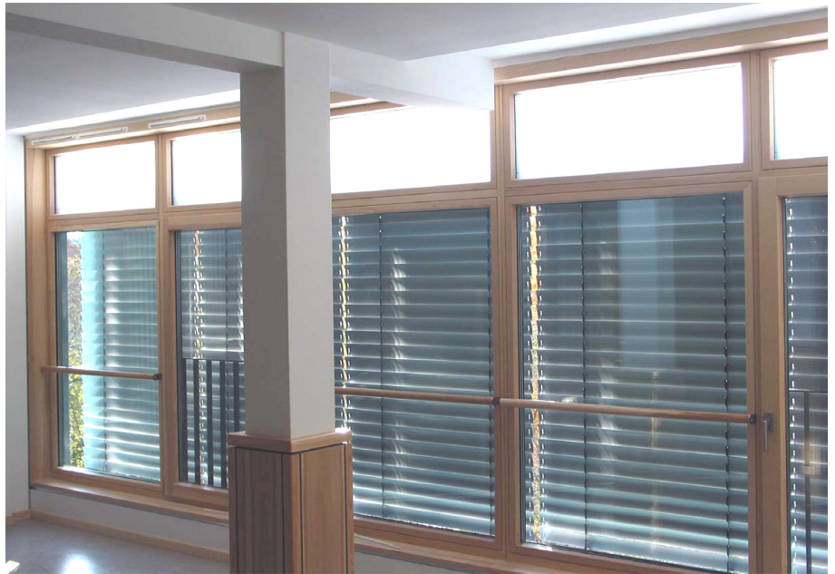
Photo of a combination of blinds with daylight redirecting glazing.
