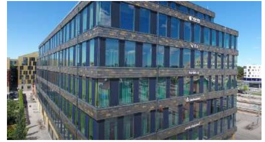
BIPV on building facade
