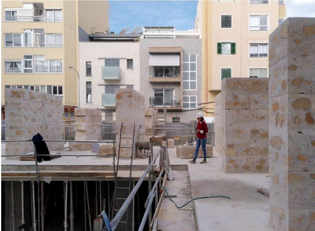
25 Temporary cohousing units, 3rd Lope de Vega st. Palma.
