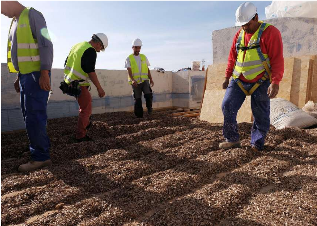
14 PPH Formentera/ Posidonia insulation, density 185 kg/m 3
