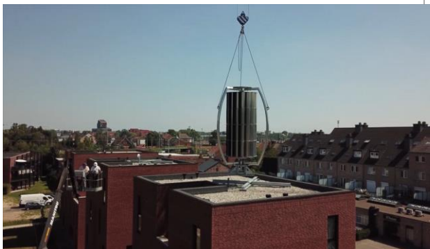
Rooftop wind turbine in residential building Source: [EXCESS project 2021]
