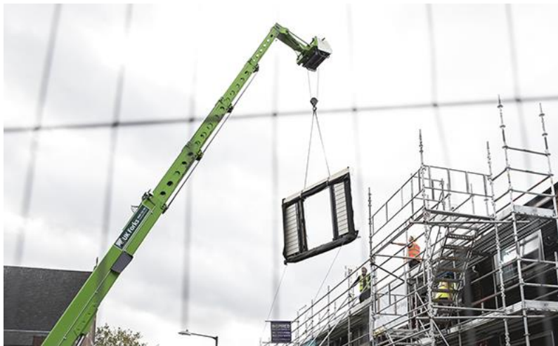
Figure 14: Installation of premanufactured facade in an Energiesprong project in the United Kingdom
