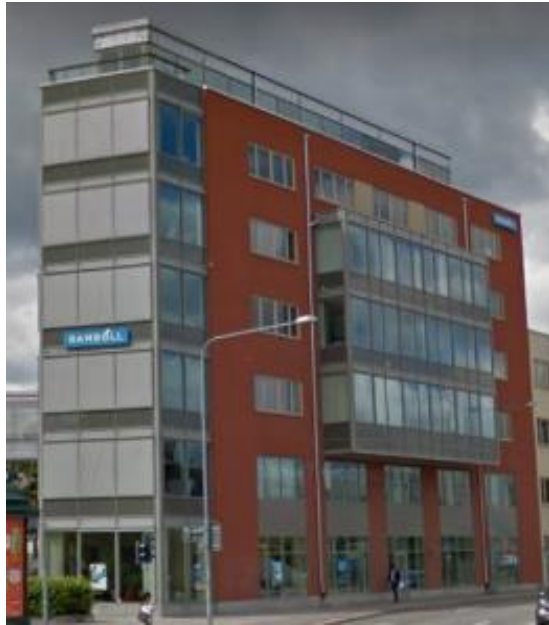
Uppsala (SWE) Vasakronan Building
