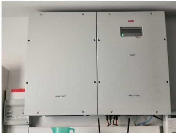
Figure 12: ABB REACT+ for electric storage installed in both villas
