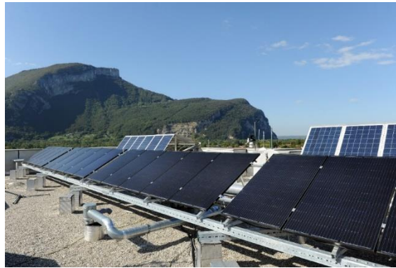
Figure 8: View of Spring 310M modules developed by DUALSUN, installed on the roof of the building
