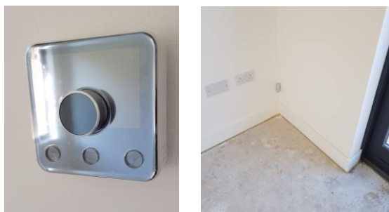
Figure 16: HIVE smart learning thermostat and occupancy detector
