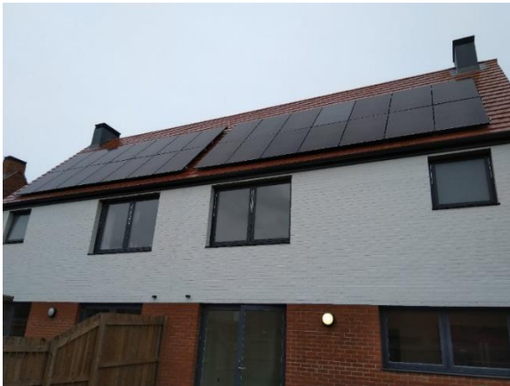
Figure 13: PV on rear (southwest facing) roof of the two semi-detached dwellings
