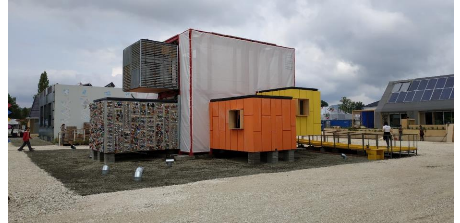
On site view of the Case Study.
