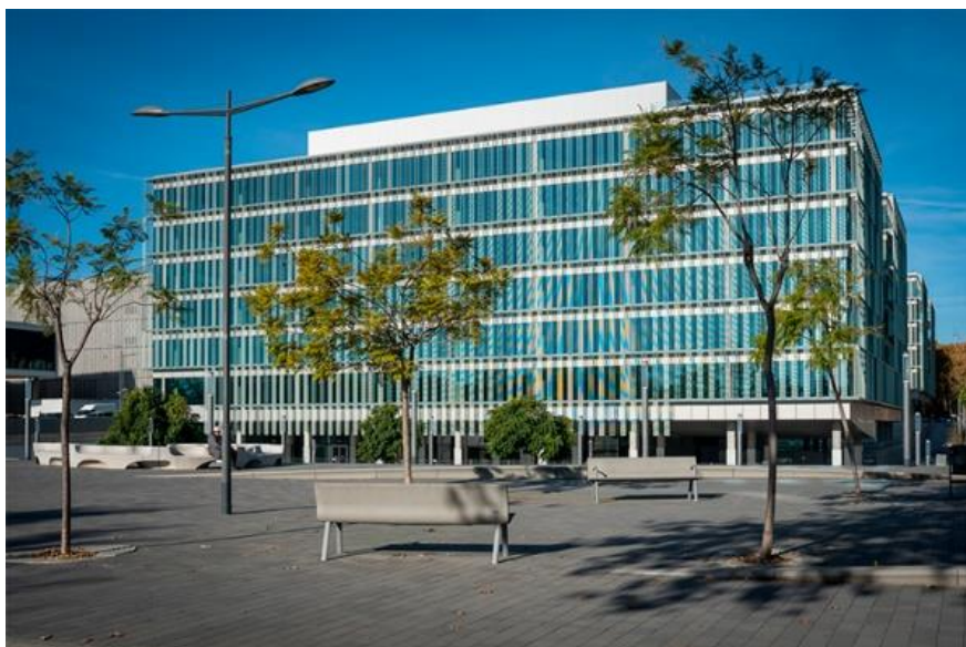
Figure 3. Administrative District building A, Zona Franca (Barcelona)
