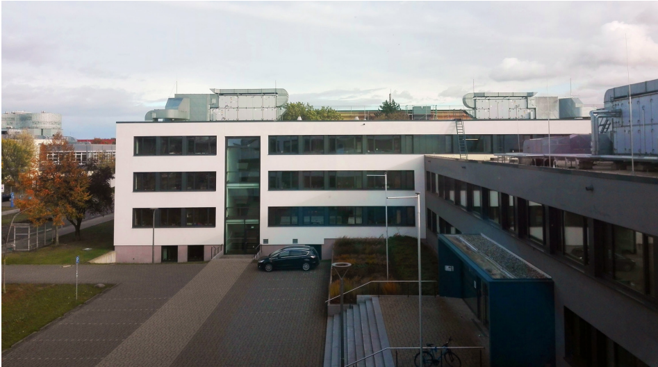
Photo 10. Max-Steenbeck-Gymnasium school building, Cottbus Source: Polish Institute of Urban and Regional Development.
