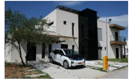
Demo site 1: nZEB Smart Home
