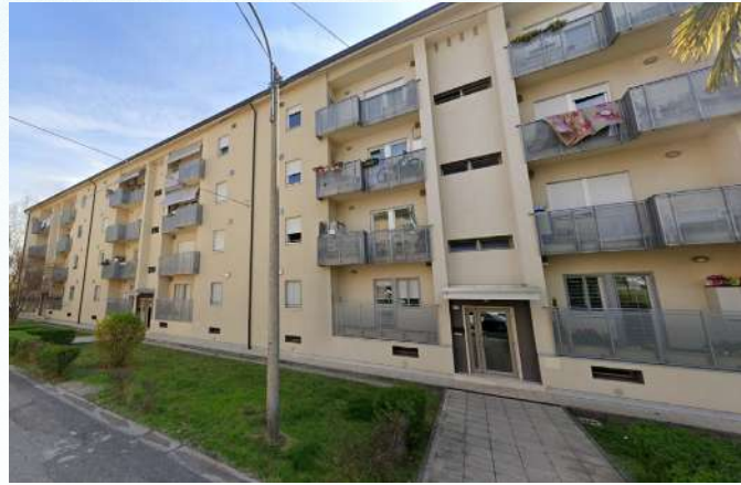
Bologna – “San Ruffillo” – Social Housing building after the refurbishment works © AESS
