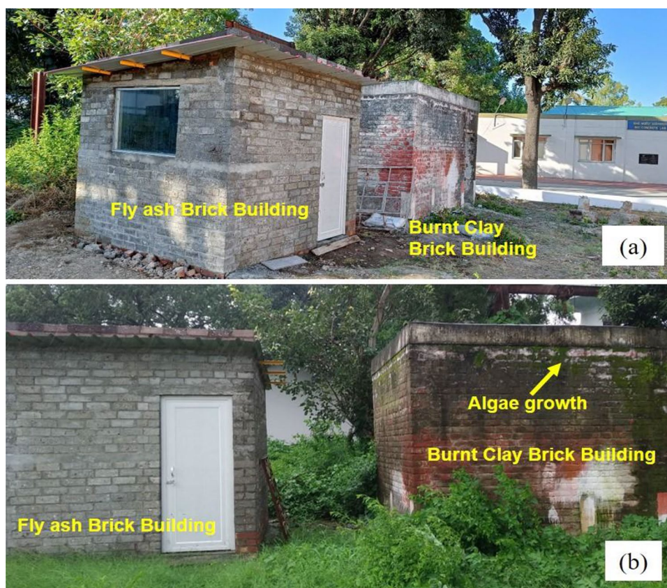
Figure 6. Physical appearance of fly ash and burnt clay bricks building during (a) Summer season, (b) Monsoon (rainy) season.
