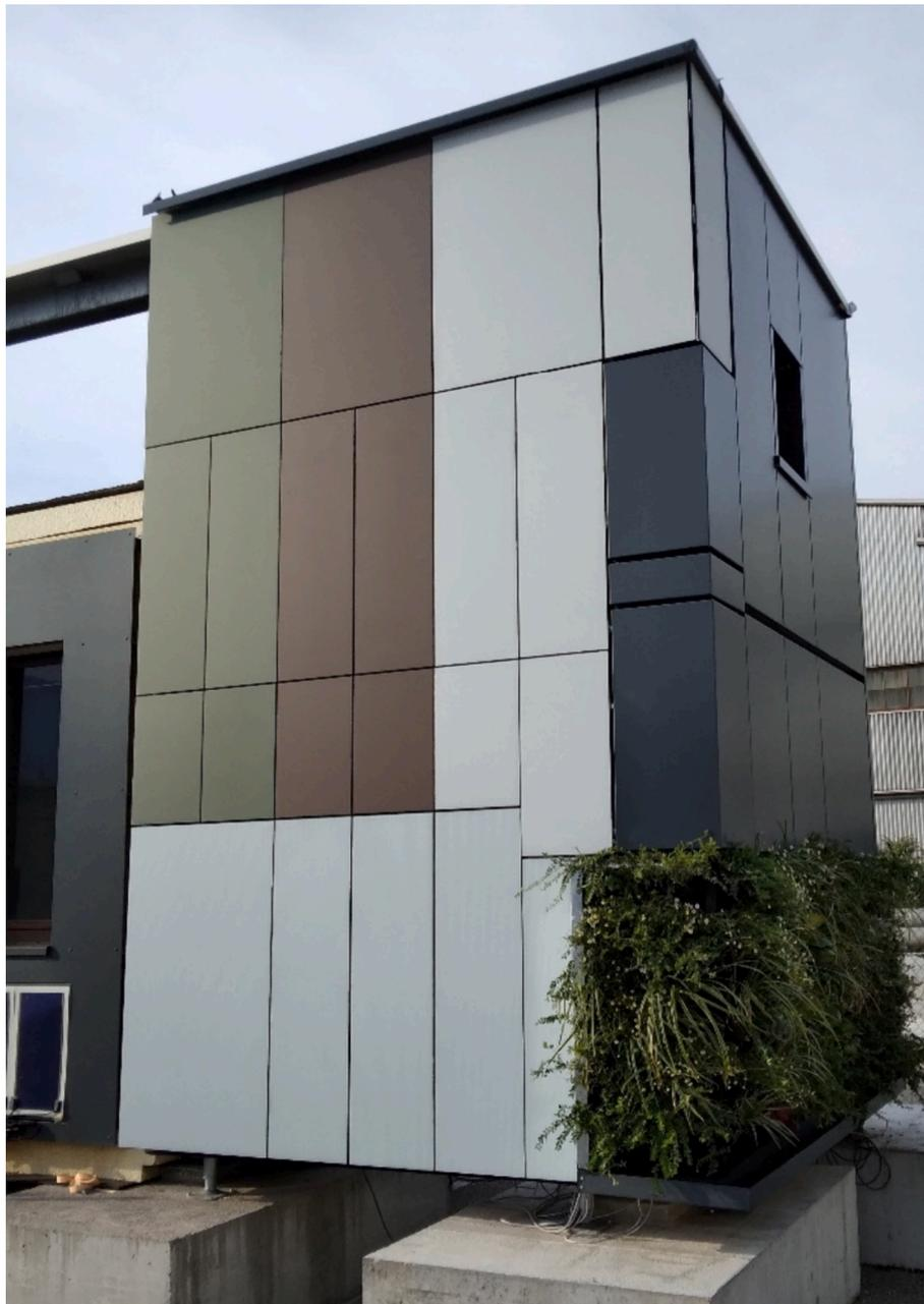
**Fig. 1.** Final layout of the Flexilab mock-up with the different multifunctional prefabricated façade cladding (i) BIPV, (ii) BIST (building integrated solar thermal) in black, and (iii) GREEN (bottom right). (For interpretation of the references to color in this figure legend, the reader is referred to the web version of this article.)
