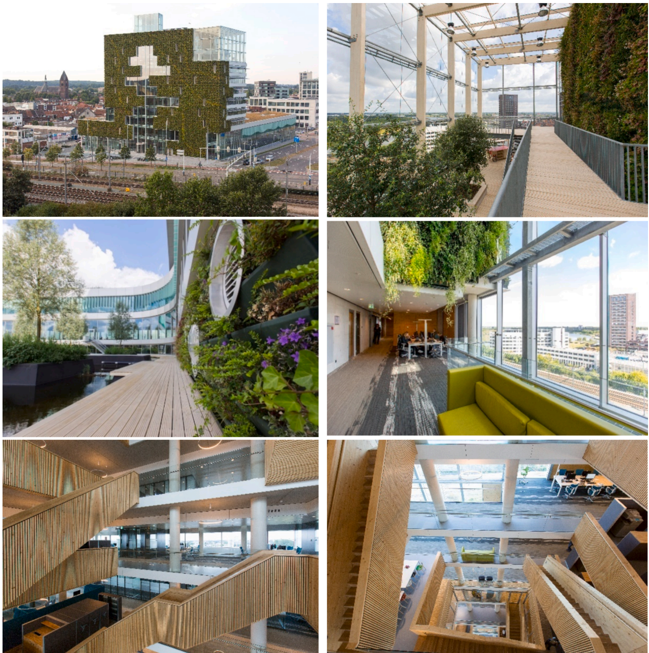
Fig. 4. Photos from the completed Venlo city hall. Image . Source: C2C Venlo. Used with permission. https://c2cvenlo.nl/media/
