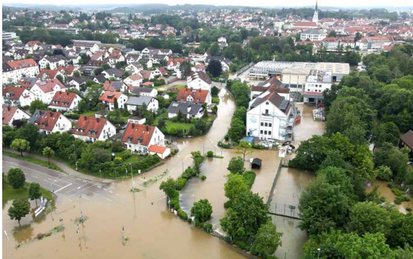
Pfaffenhofen Ilm, Germany was severely affected by floods in 2024/Shutterstock
