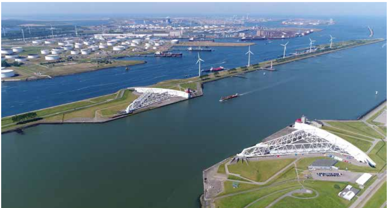
Storm surge barrier, Rotterdam, Netherlands © Shutterstock
