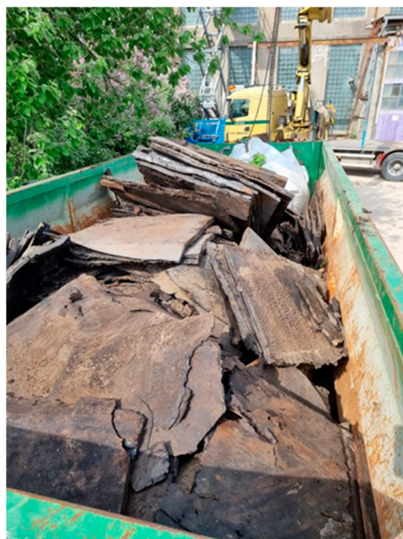
Figure 1. BBRM waste from a demolition site.
