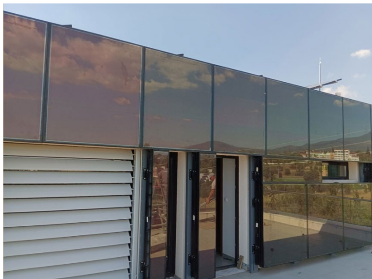
Fig. 2. Manifested Adaptable dynamic building Envelope system (source: CERTH)
