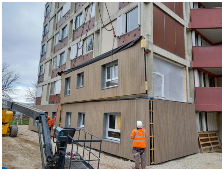
Fig. 5. Fixing PanoRen panels to a wall (source: rehouse-project.eu)
