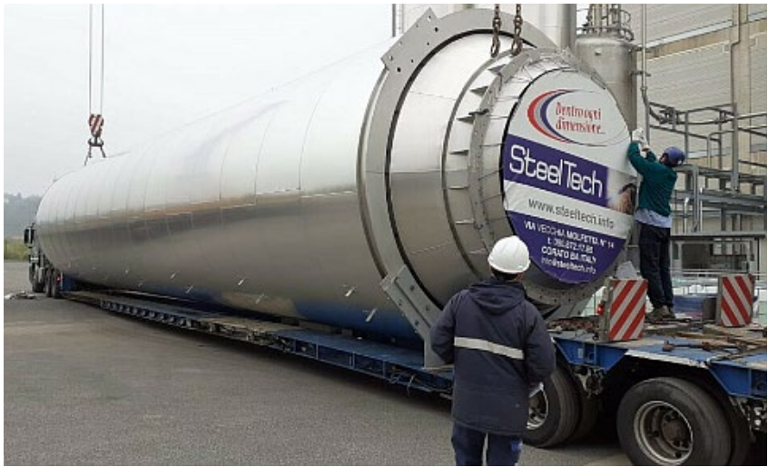
Fig. 4. Energy storage tank of a centralized holistic renovation kit (source: rehouse-project.eu)
