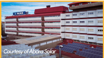
Zaragoza’s hospital: High heating needs (2023, ES)
