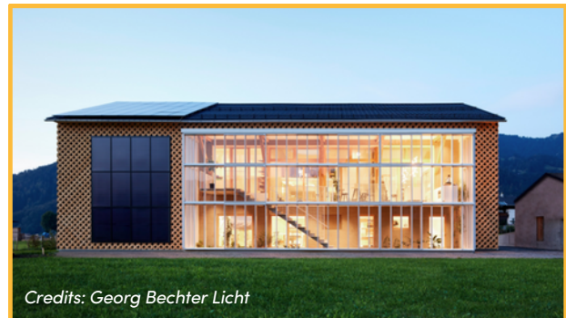
GEORG BECHTER LICHT think tank – Solar thermal, PV and heat pump hybridization
